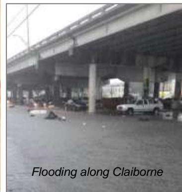
The recent flooding along Claiborne has confirmed data developed by the City and the Trust for Public Land. According to their maps, I-10 is a primary contributor of large amounts of stormwater run-off in the corridor. The land below the highway is paved, making the area highly impervious. Additionally, subsidence has caused depressions and low points that worsen
